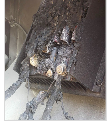
Burnt Battery equalizer from bus fire
