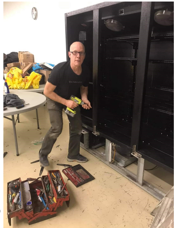
Lloyd putting the doors back on the newly purchased fridge unit at the Blessing Centre in Brantford
