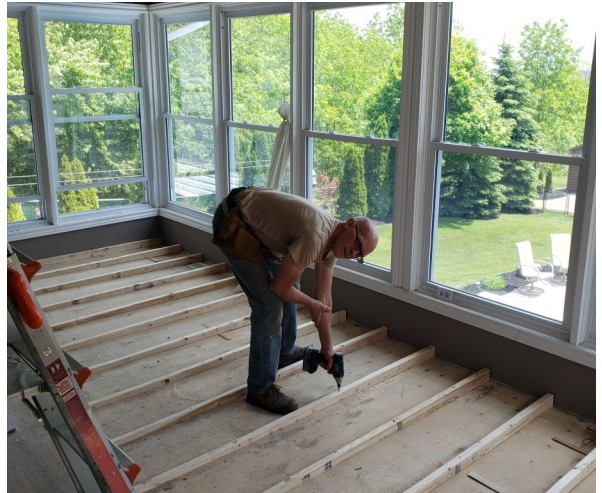
Lloyd working a job that's different because of the loss of ability to travel. Lloyd is currently working for a renovation company and other jobs to make up for lost income.
